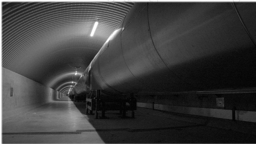
FIGURE 6 View of the vacuum-sealed tube inside Virgo's West Arm, November 2025
